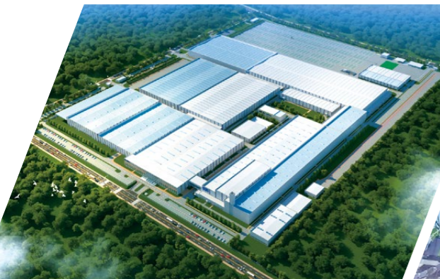
CHANGAN Automobile Thailand Manufacturing Construction Project
