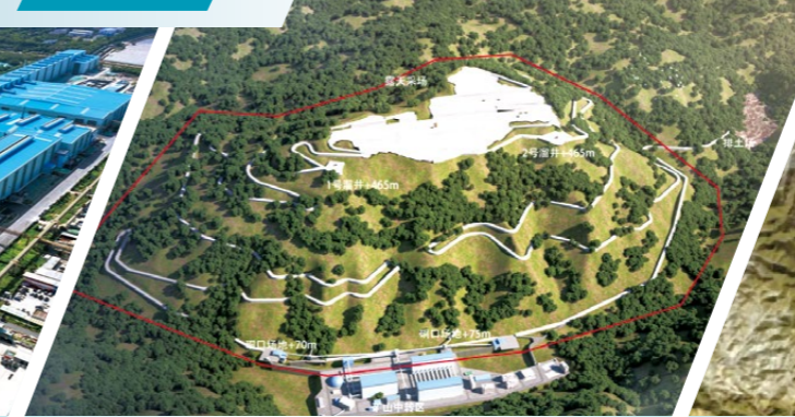
Huangshi Yuntoudao Limestone Mine Project
