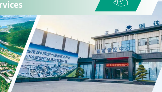
Lianyungang Yaxin Steel Intelligent Factory Project
