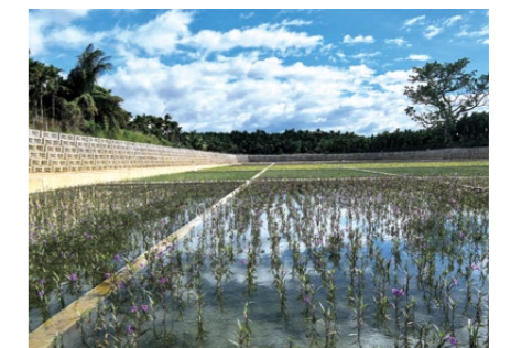
Nanfeng Creek Water Environment Improvement and Aquatic Ecological Restoration Project
