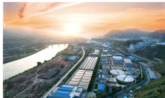
Lanzhou Yanerwan Sewage Treatment Plant
