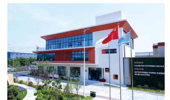
Fully Prefabricated Steel Structure R&D Building
