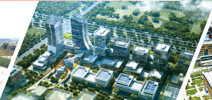
Infrastructure Pipeline Network Project for the CEEC Bazhou Zhigu Industrial Park
