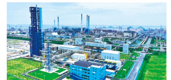
Hydrogen-Based Shaft Furnace Project
